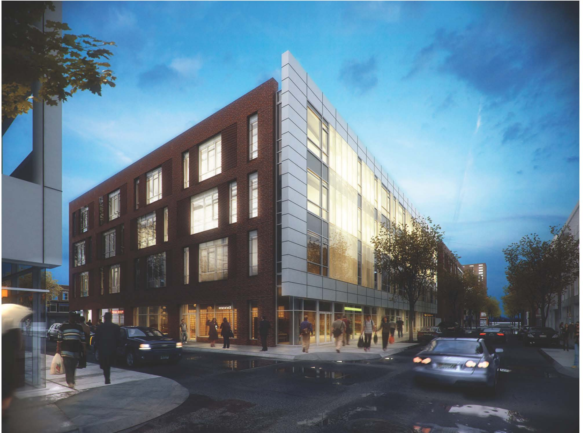
William Street Southeast View (Building 2 )
