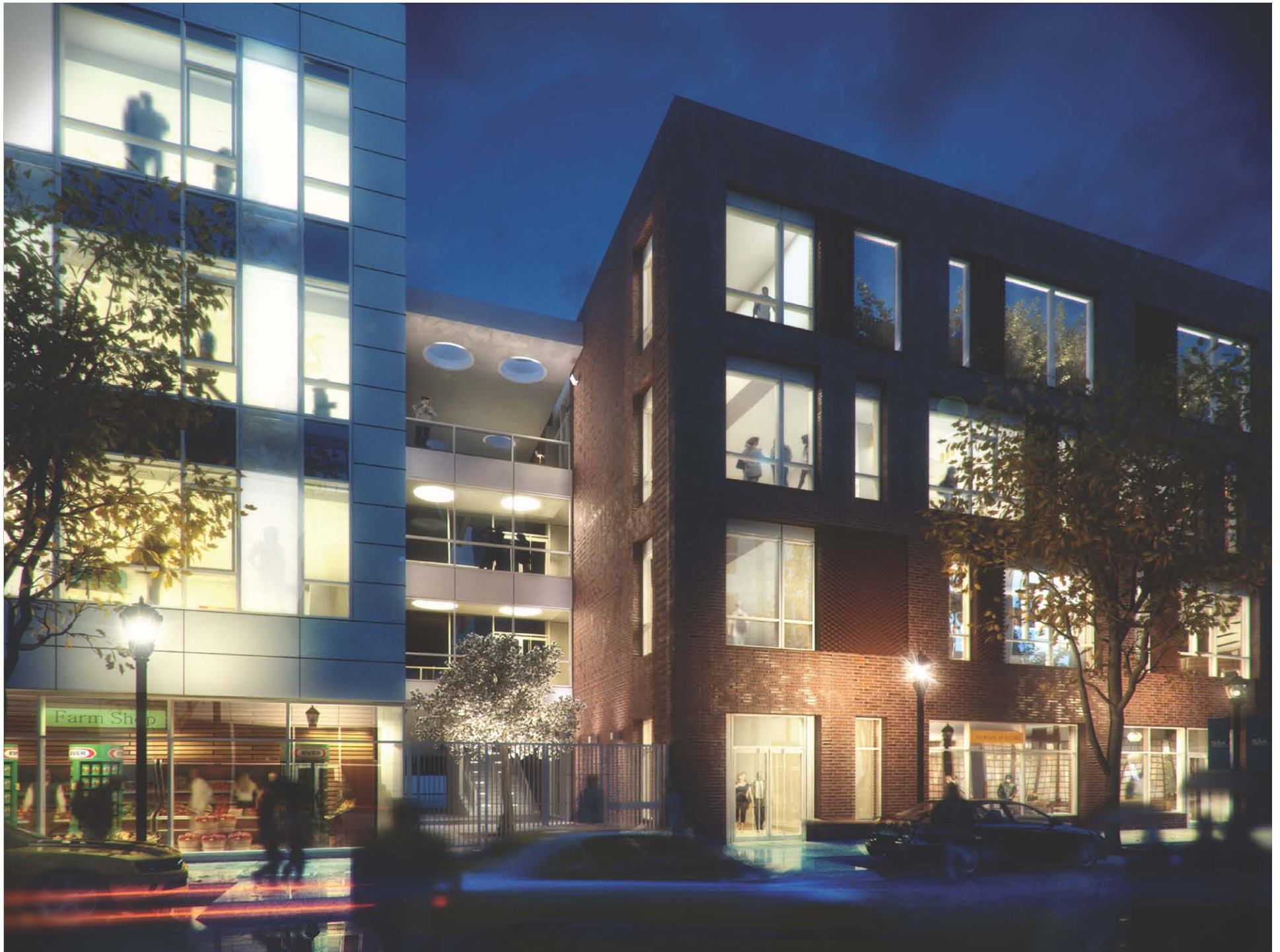
Halsey Street Southeast View (Building 2 )
