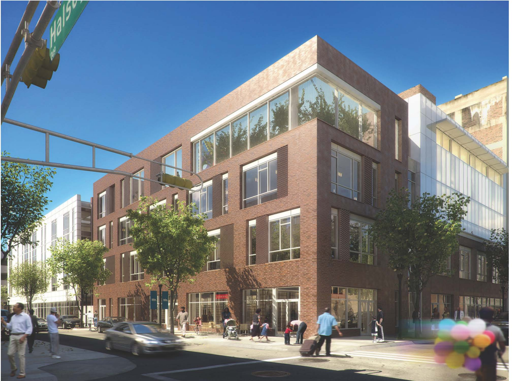
240 Halsey Street (Building 2 )
