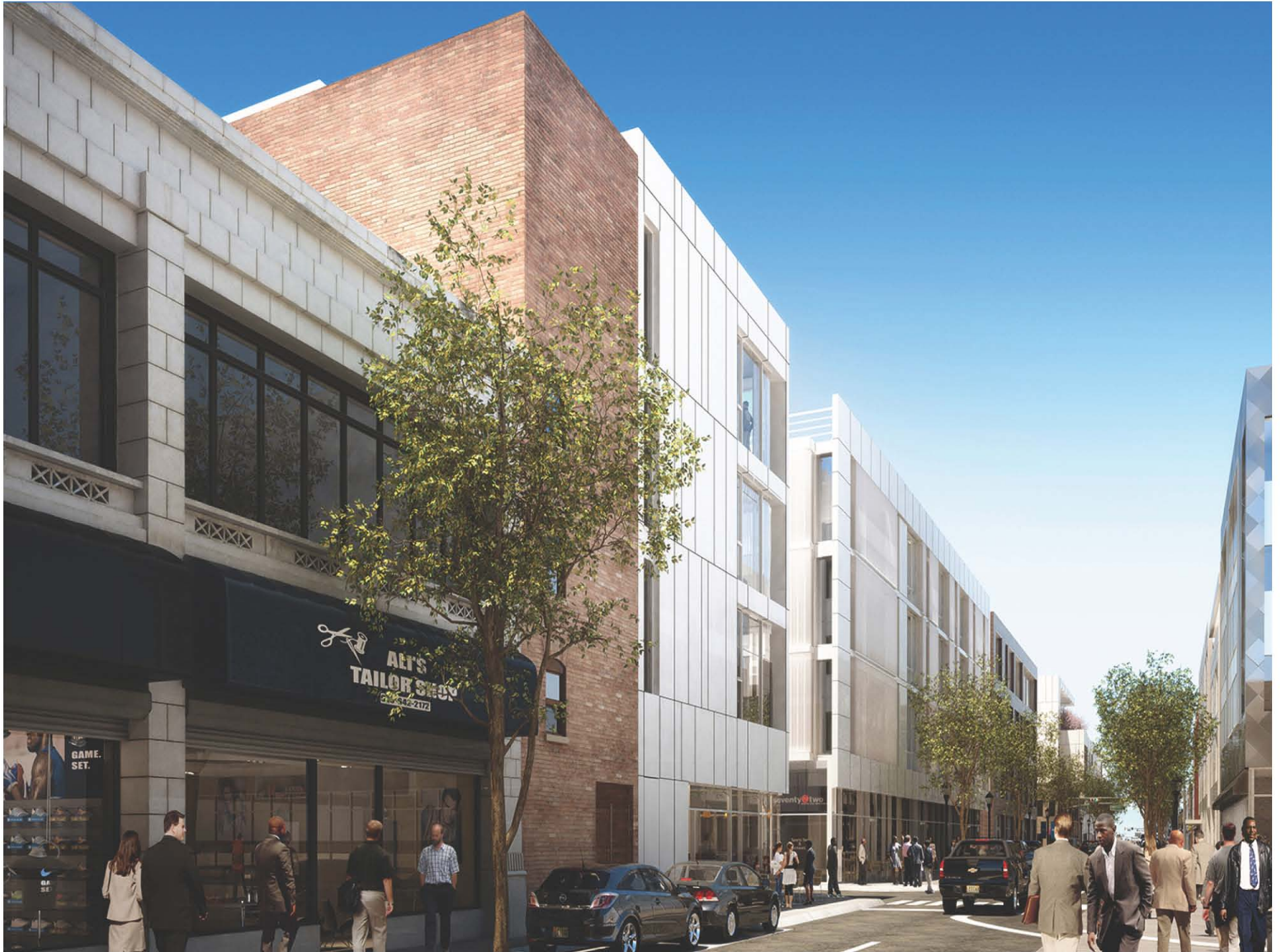
William Street East View
